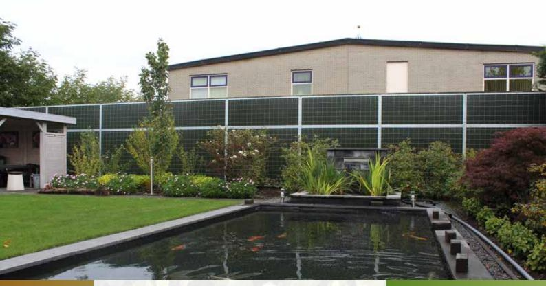
The Noise-Reducer® Noise Barrier is a lightweight construction with high insulation and absorption properties. On either the noise-side or on both sides of the panel a galvanised steel wire-net and a polyethylene separator-net secures a layer of high absorptive mineral wool.
