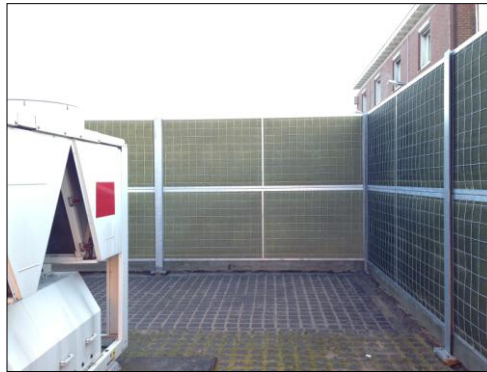
Noiseside: Mineral wool and nettings Backside: coated steel plate
